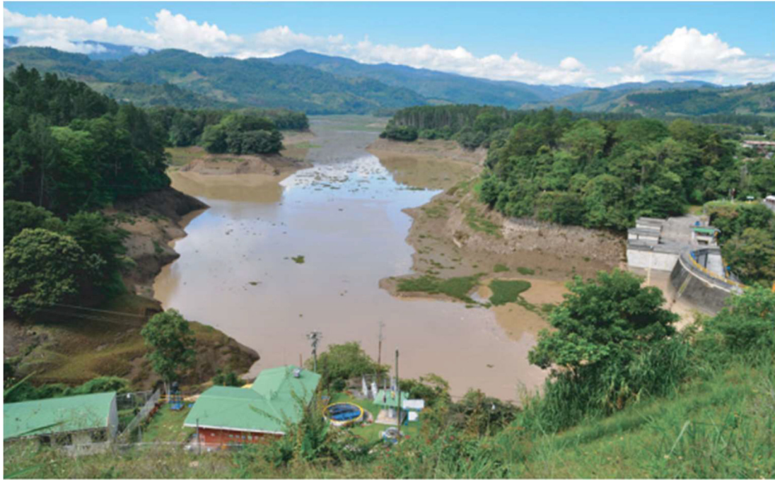
Fig. 6. Combination of factors like turbidity current, delta propagation, and sediment production from riverbanks causes sedimentation in Cachi reservoir, Costa Rica [33].
